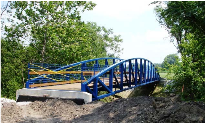
The bridge was set in place by a 165 ton crane and secured in less than 30 minutes.
